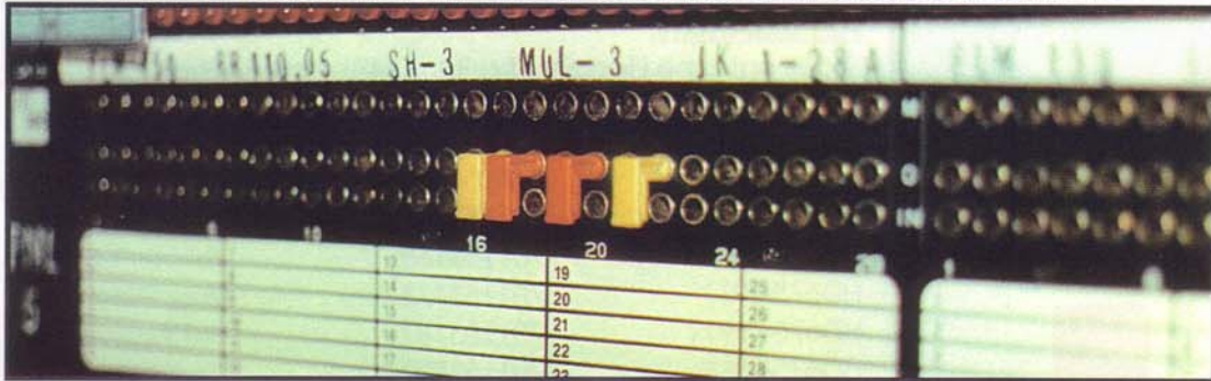
BANTAM DSX PANEL WITH I.D. PLUGS & 1.544 I.D. CAPS INSTALLED
